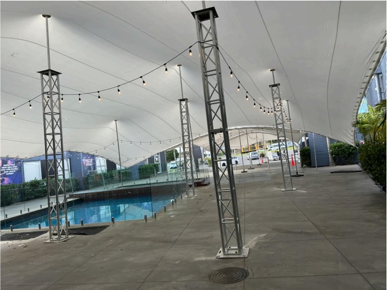
16 x 18m & 10 x 20m Joined Canopy with Truss king posts and festoons
